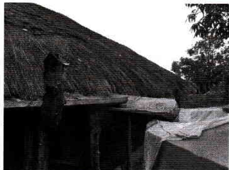
Figure 6 Collecting water from thatch with wooden gutters
