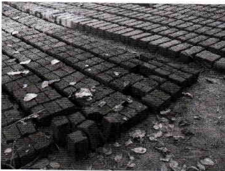
Figure 1 The clay blocks for the formwork
