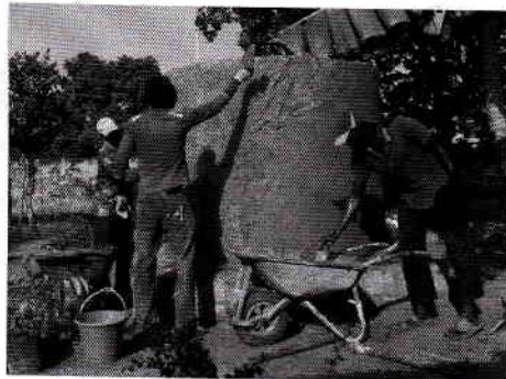
Figure 2 Tank under construction: the first layer of mortar is applied
