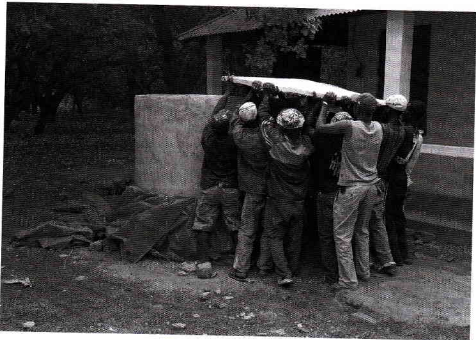
Figure 3 Lifting the tank cover on to the tank
